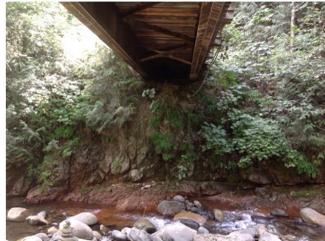
Right Bank Abutment when facing downstream
