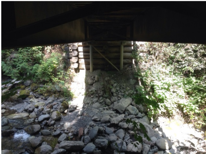
Left Bank Abutment when facing downstream
